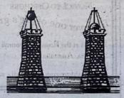
accurate timepiece recording the time at port at some known longitude. As ships prepared to depart Port Phillip they could set the ship's chronometer precisely to Melbourne time by keeping a watch on the timeball. At exactly 1 p.m. each day the ball would be dropped from its elevated position
